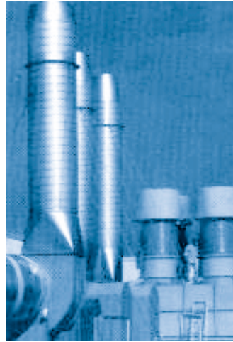
Four low-profile BS-5 Tri-Stack systems provide 40,000 CFM each; their counterpart belt-driven centrifugal fans on the left are more than twice as tall.
