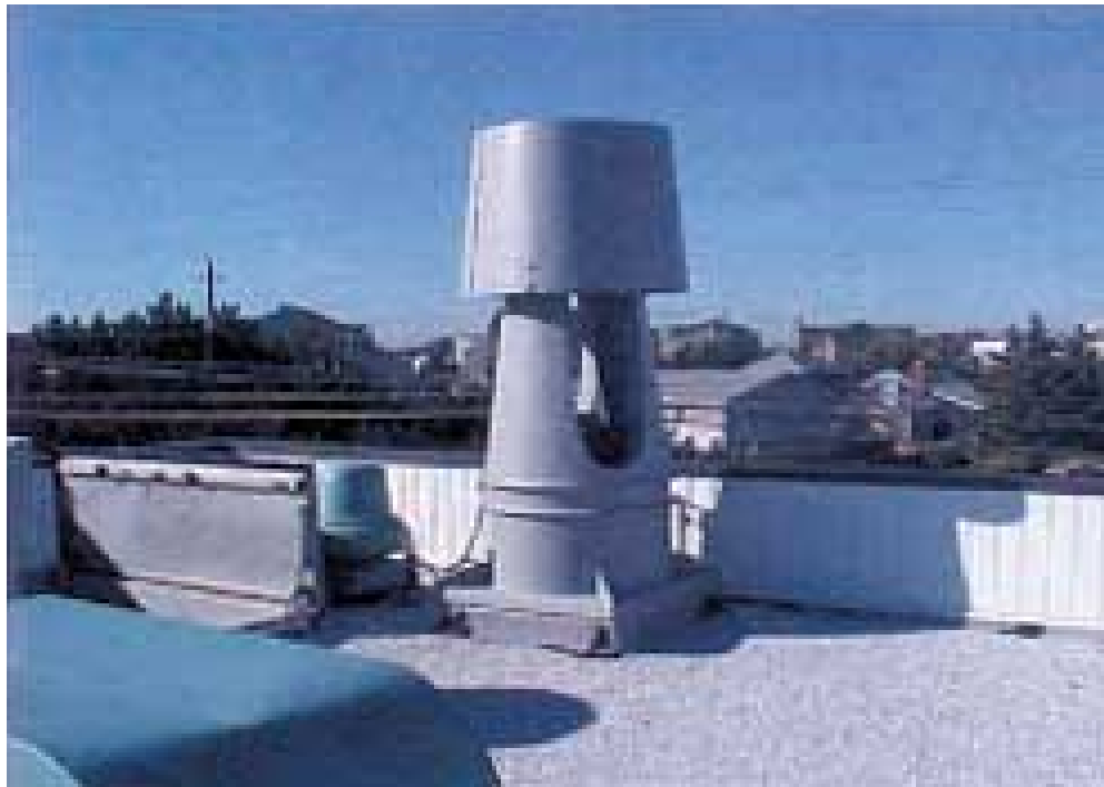
Mixed flow stacks are substantially shorter and have less visual impact.
